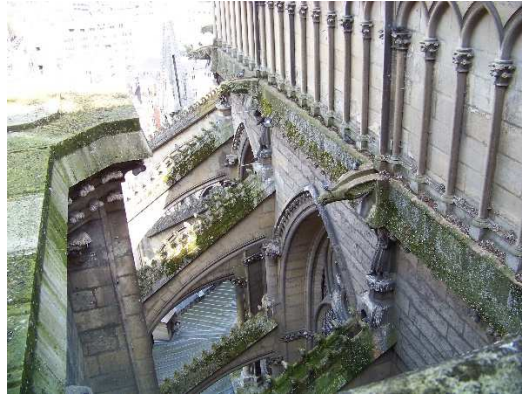
Fig. 1: Photo of the Rheims cathedral apse made of the Courville and Ditrupa stones in wall elevations and Savonnières stone in caps and decorations of buttresses (photo: G. Fronteau 2008).
