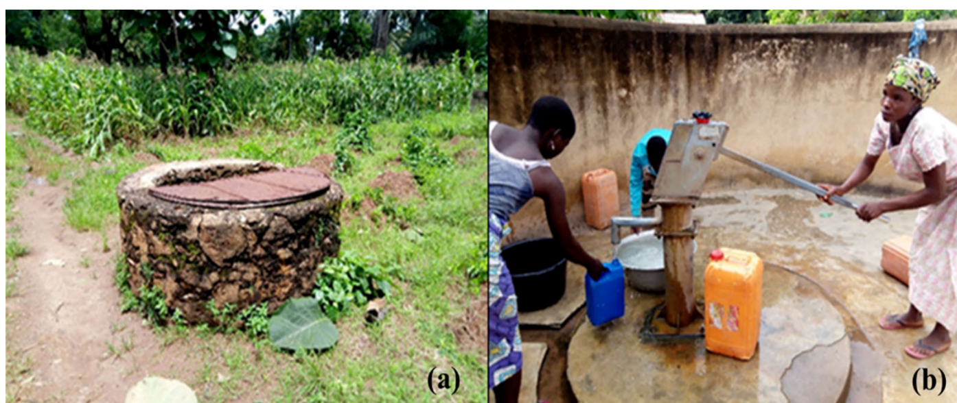
Figure 4. Traditional sinks exploiting the water of the alterite reservoir at Niamtougou (northwest of the study zone) (a) and borehole equipped with a human-operated pump, exploiting the water of the fractured reservoir at Bébéda (center of the study zone) (b).
