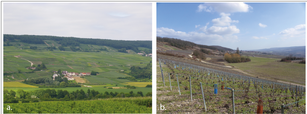
Figure 4. The Jacotines landslide from the opposite valley side (a) and side view of the head scarp (b).
