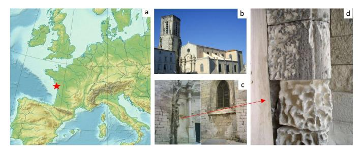
**Figure 1.** (**a**) La Rochelle location in western France; (**b**) Saint Sauveur Church; (**c**) walls and columns showing severe weathering; (**d**) detail of black crusts and alveolizations on one column. Red Star: La Rochelle location.
